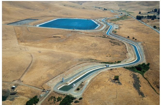
Aerial view of the South Bay Aqueduct and Dyer Reservoir. Credit: Department of Water Resources
