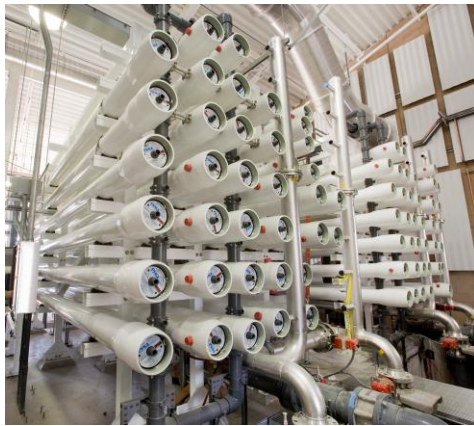
Reverse Osmosis membranes – similar to those at Zone 7's Mocho Demineralization Facility – would provide highly treated recycled water for injection into the Main Basin.
