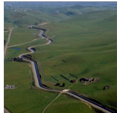
Supply from the SWP is delivered via the SBA. Approximately 90% of Zone 7's existing supply is conveyed through the SBA.
