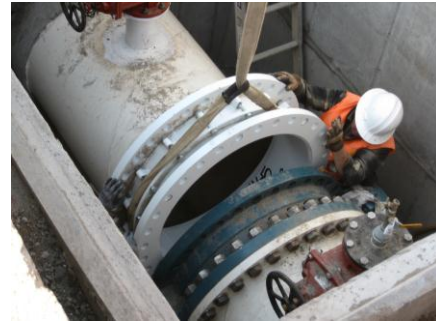
Construction of El Charro Pipeline in 2009
