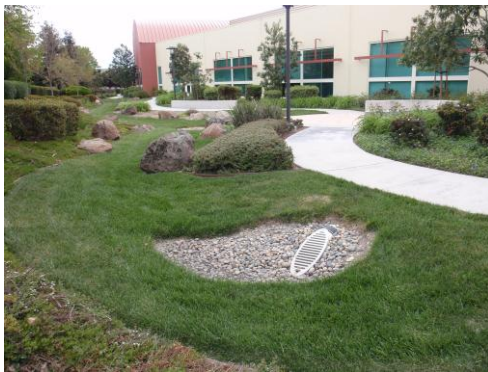
Drain rock is used to prevent erosion of this vegetated swale at Zone 7 Water Agency's office building – drain rock can also enhance recharge if placed over permeable areas of the groundwater basin.
