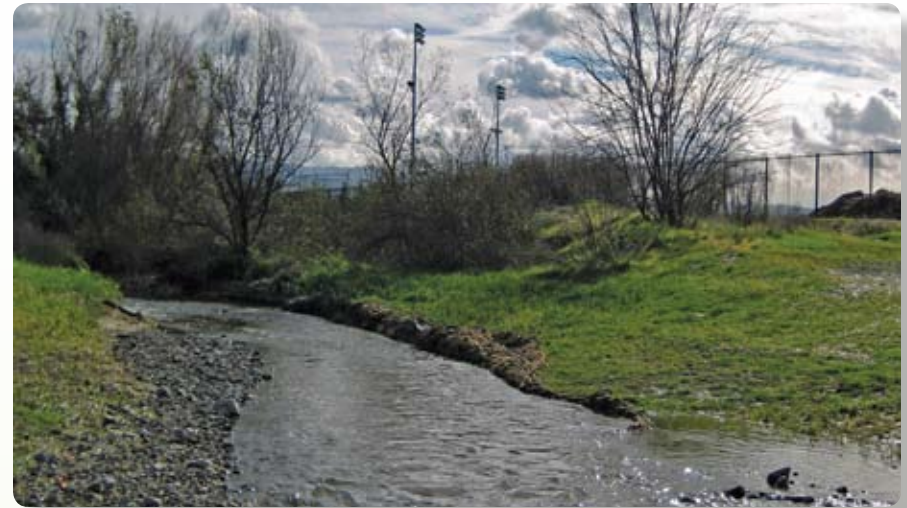
Removal of a concrete crossing of Arroyo Mochó in Livermore exemplifies the StreamWISE vision.
