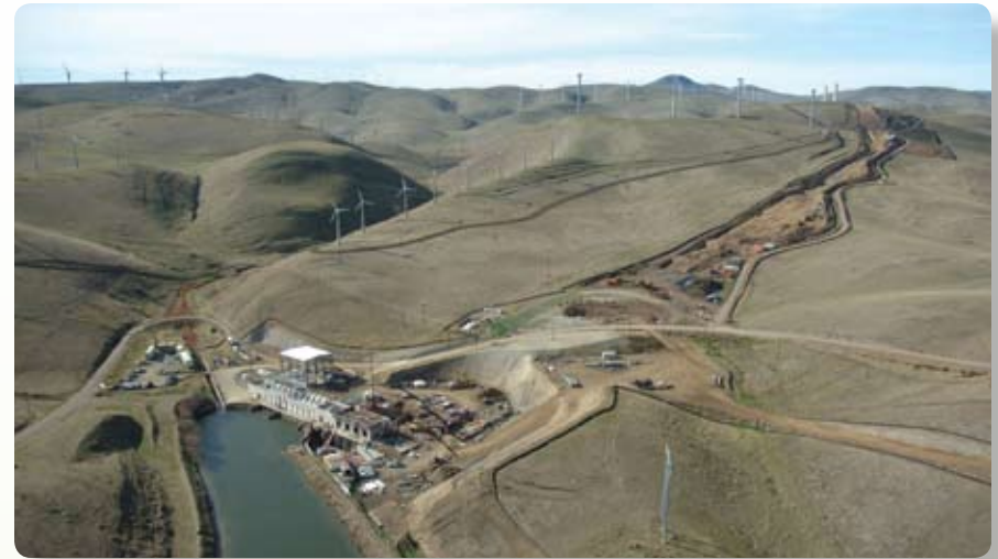
State Water Project's South Bay Aqueduct is being improved and enlarged.
