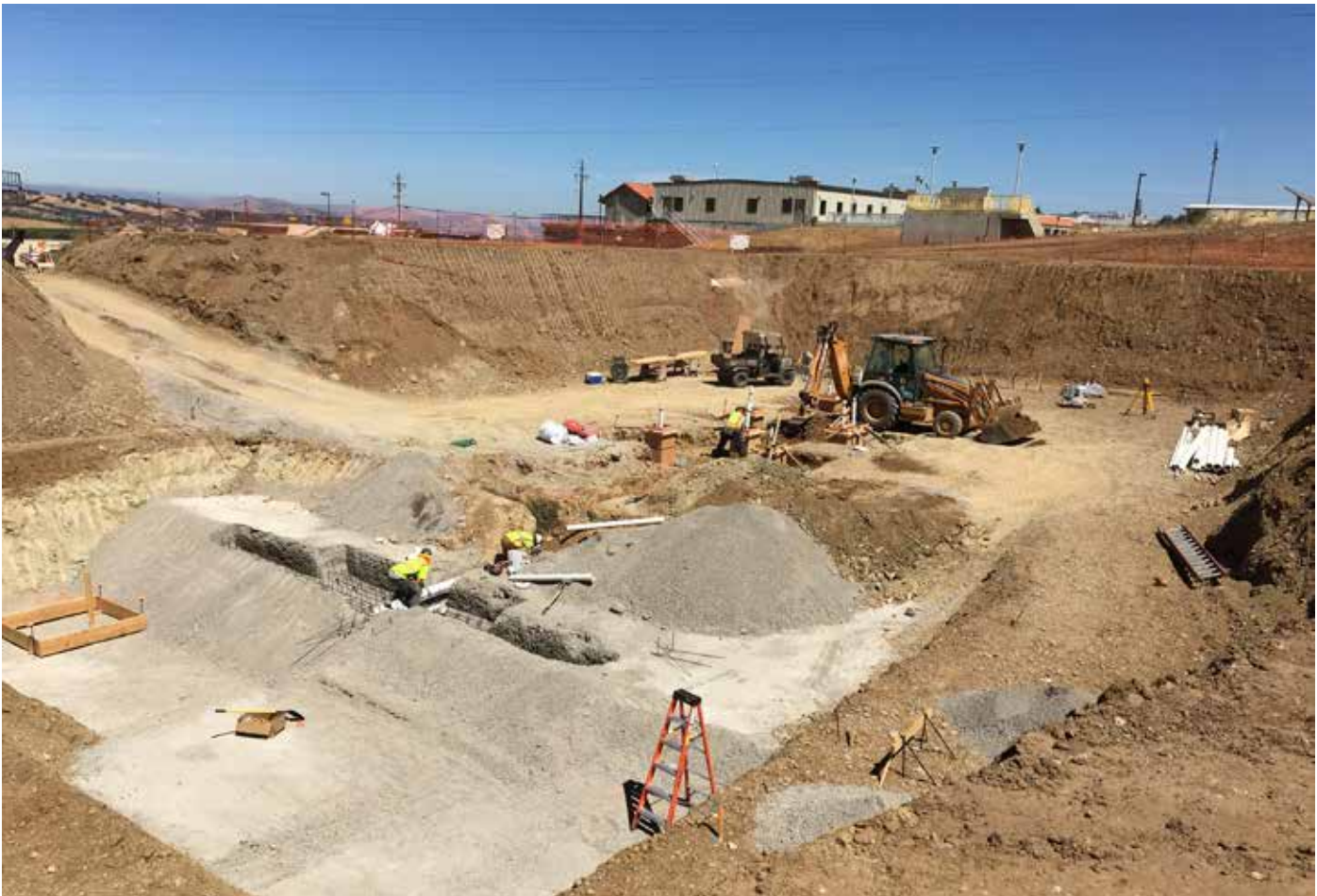
Del Valle Water Treatment Plant Ozone Project
