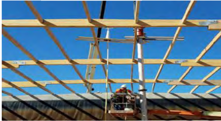
DVWTP 3 MG Clearwell Roof
