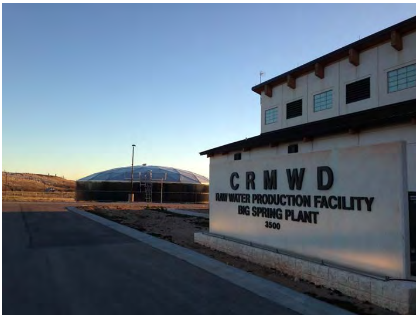
Figure 2.7 Colorado River Municipal Water District's Raw Water Production Facility in Big Spring, TX
