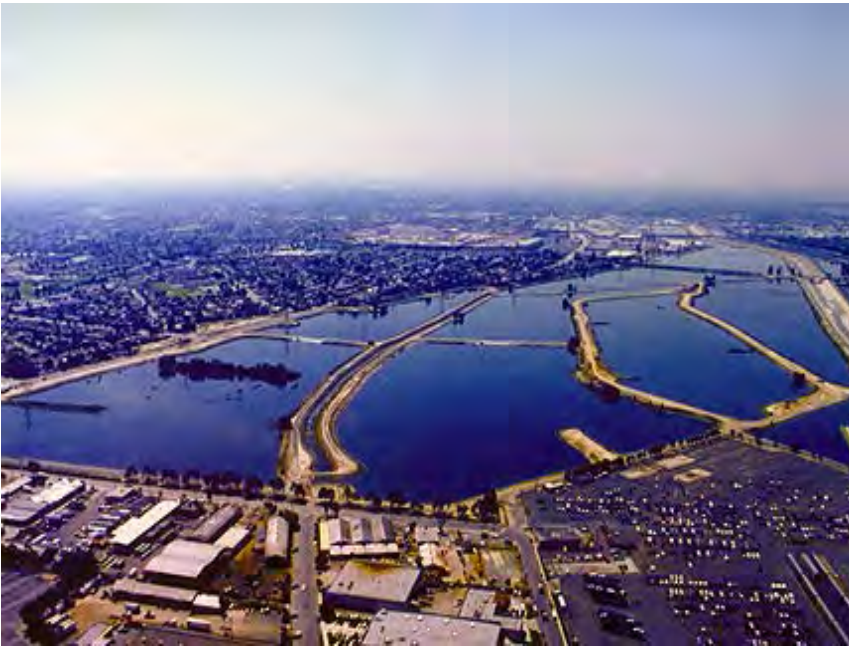
Figure 2.4 Rio Hondo Spreading Grounds
