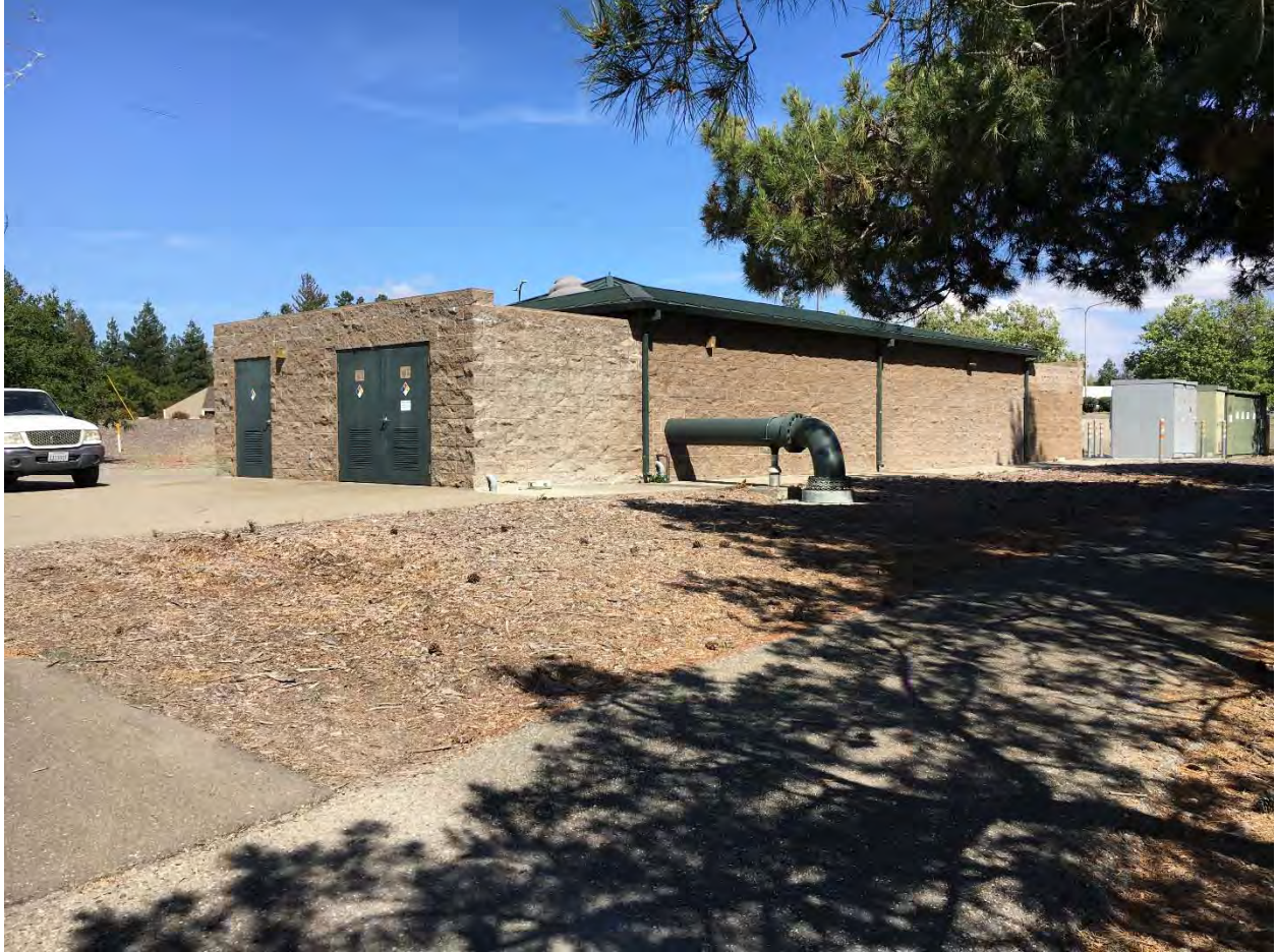
Figure 8 View of Zone 7 Chemical Building from West Side of Site
