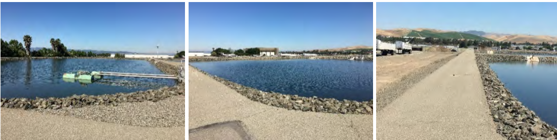
Figure 7.4 Abandoned Facultative Sludge Lagoons
