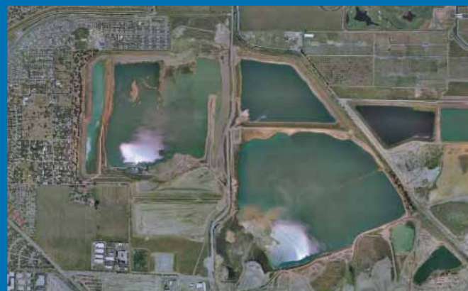
Zone 7 will reduce peak flows in Arroyo Mocho and Arroyo las Positas by diverting excess water into the future Chain of Lakes for storage. Stormwaters will be detained in the Chain of Lakes until peak flows have subsided, then released back to the arroyos in a controlled manner.
