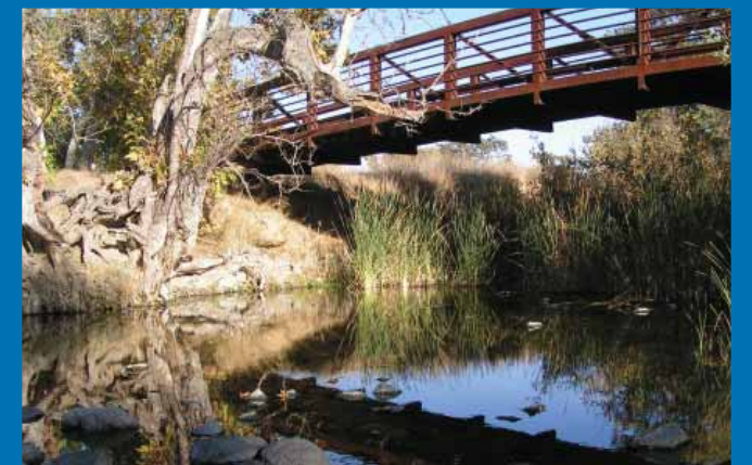
A walking bridge crosses Arroyo del Valle in Sycamore Grove Park enhances quality of life for the community.
