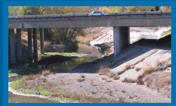
Sedimentation buildup, as shown here at the confluence of Arroyo del Valle and Arroyo de la Laguna under Interstate 680, can impact downstream areas.
