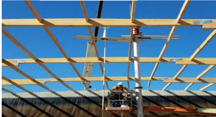
DVWTP 3 MG Clearwell Roof
