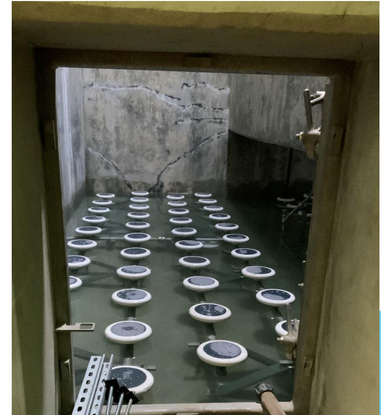
Testing Diffusers for Leaks – 12/28/21
