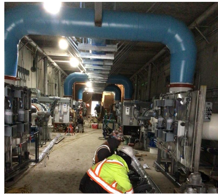
General View of Pipe Gallery – 12/29/21
