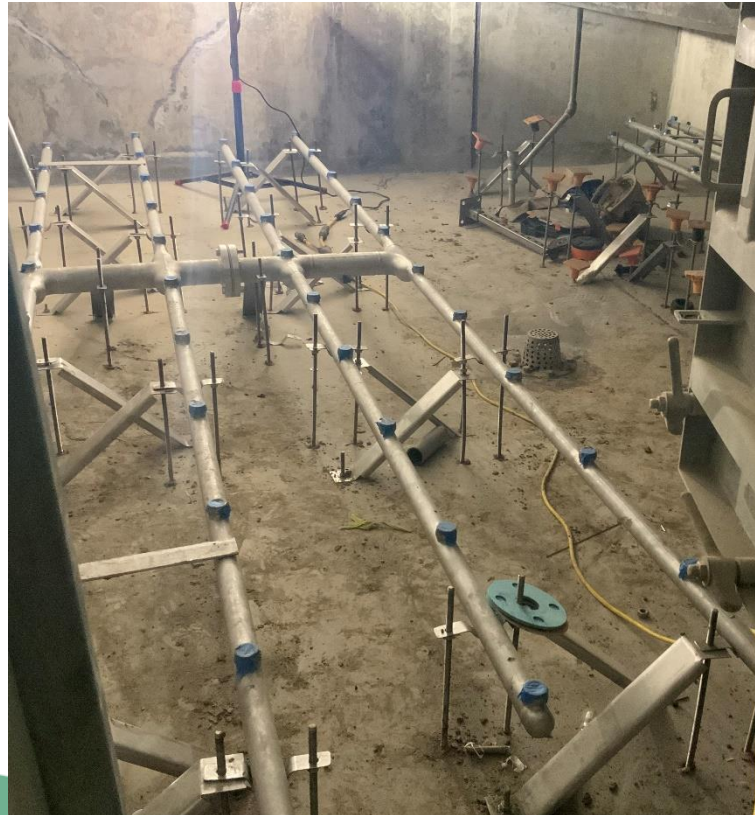
Installing Diffuser Piping Manifolds – 12/15/21
