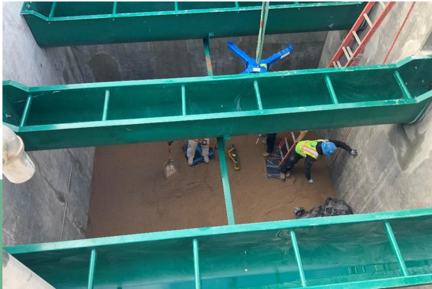
Installing Sand Filter Media – 12/15/21
