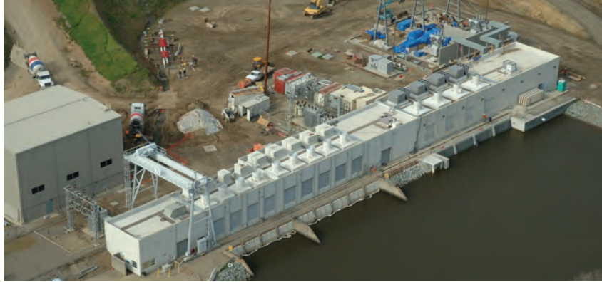
DWR's South Bay Pumping Plant Stage 3 expansion was completed in January 2010.
