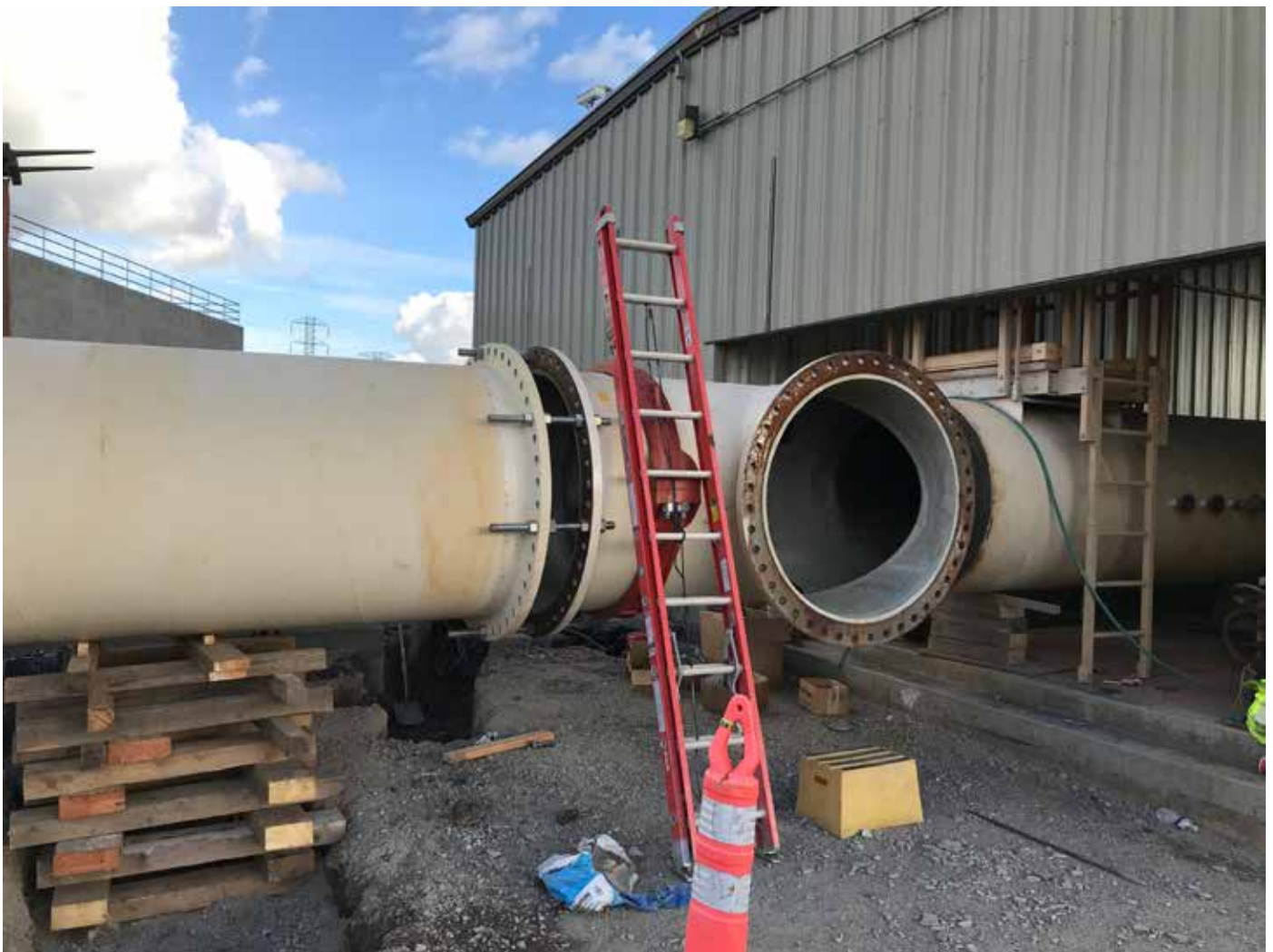
Del Valle Water Treatment Plant Ozone Project
