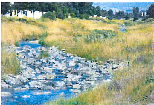
Stanley Reach - new roughened channel
