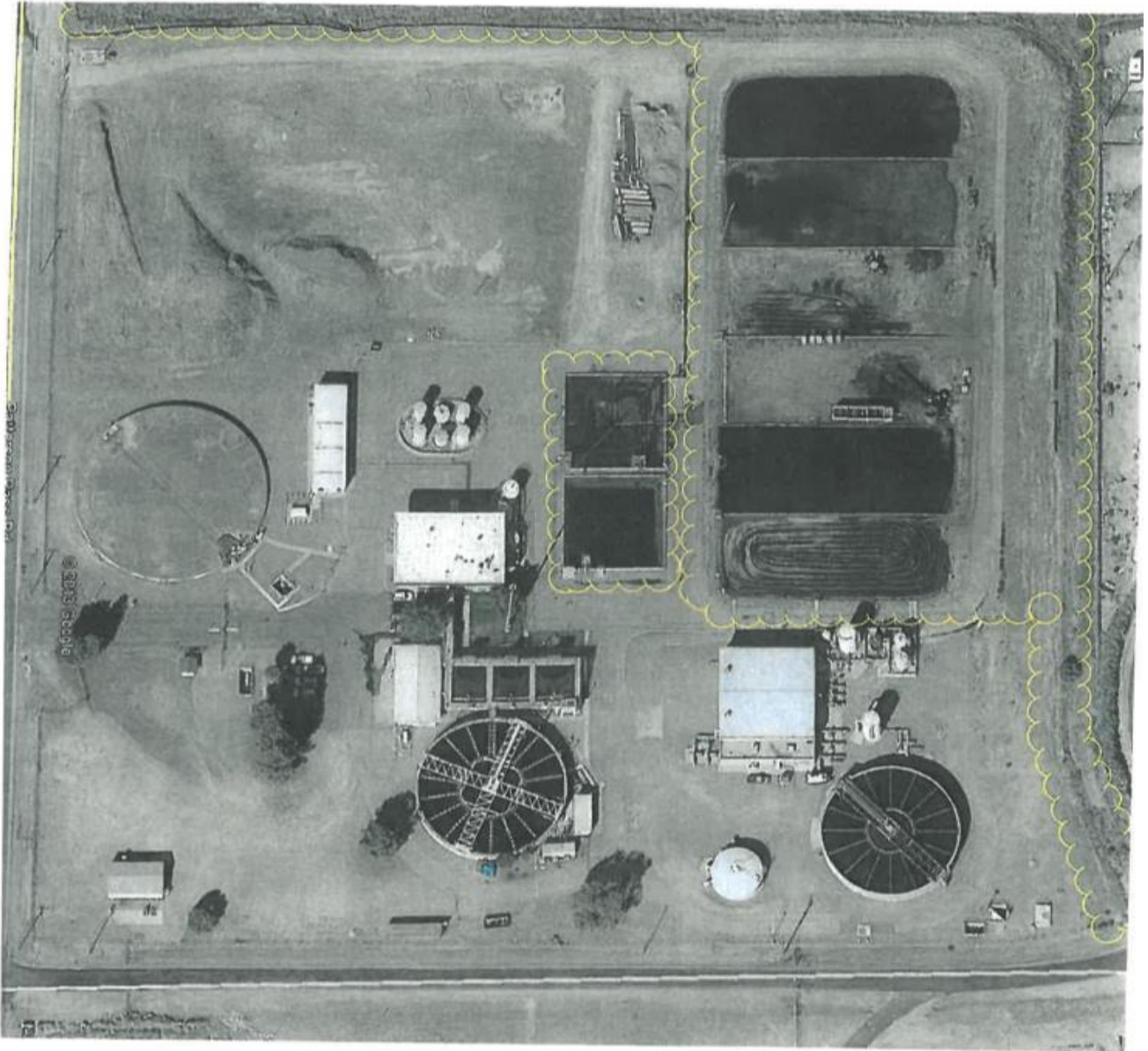
PATTERSON PASS WATER TREATMENT PLANT (NO SPRAYING OUTLINED IN YELLOW)
