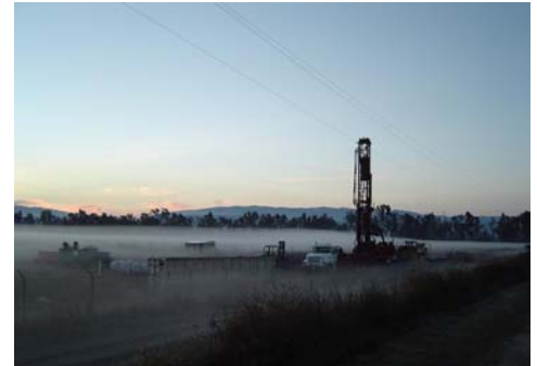
Drilling of the new wells.
