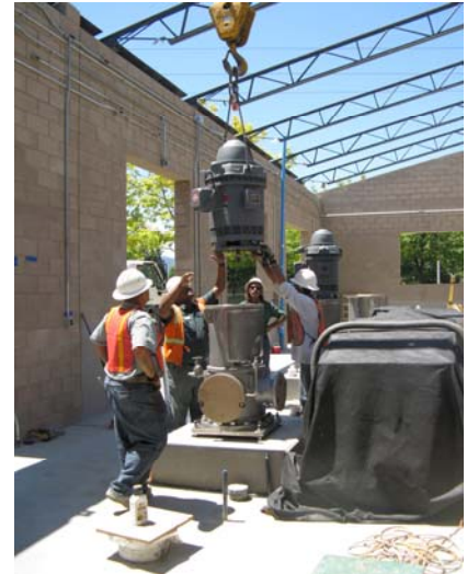
Installation of a RO feed pump.
