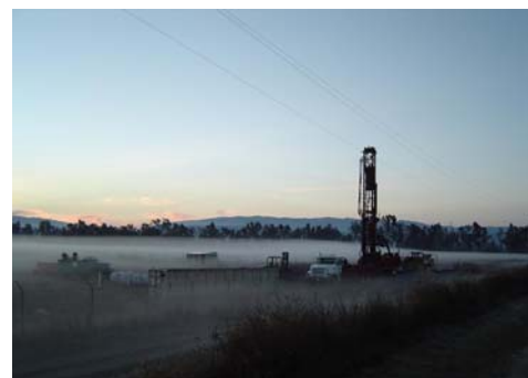
Drilling of the new wells.
