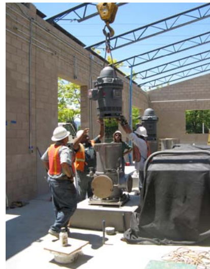
Installation of a RO feed pump.
