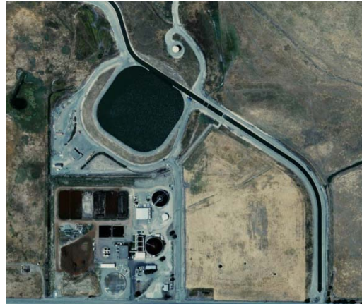
Zone 7 is evaluating the potential for either building a new water treatment plant or expanding an existing water treatment plant.
