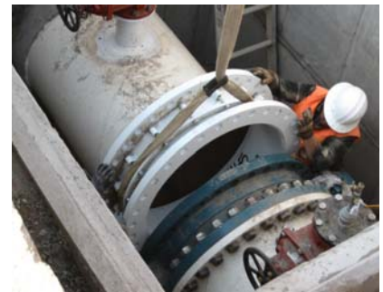
Construction of El Charro Pipeline in 2009
