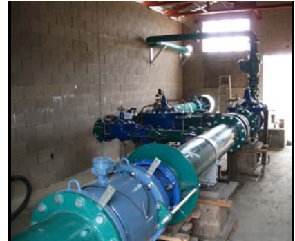
Construction of a Well at the Chain of Lakes Well Field
