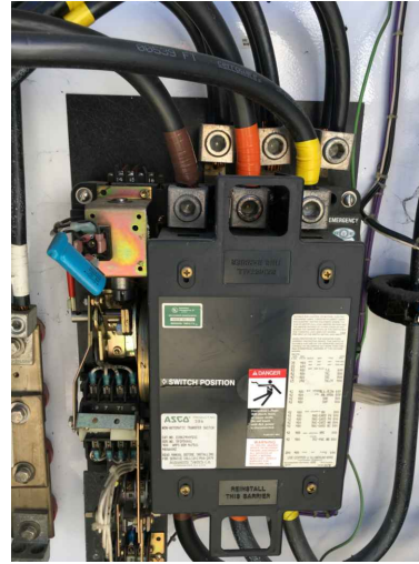
SINGLE LUGS 350 MCM ROTATION COUNTER CLOCKWISE
