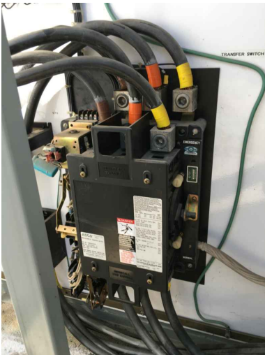
SINGLE LUGS 350 MCM ROTATION CLOCKWISE
