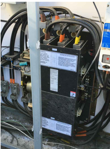
DOUBLE LUGS 4/0 ROTATION COUNTER CLOCKWISE
