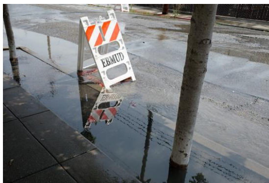
EBMUD crews set up caution signs while responding to flooding in the street
