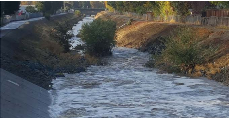
PHOTO 3: Looking downstream where the channel transitions from the concrete confluence structure to earthen trapezoidal channel.
