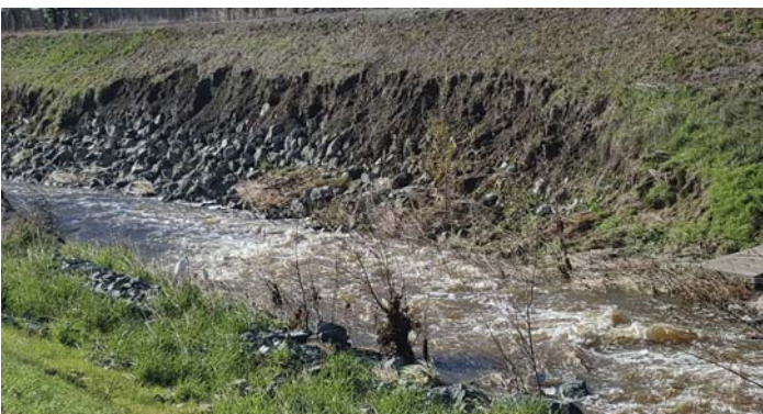
PHOTO 4: Looking at the right bank that was damaged as a result of 2017 storms and reconstructed in 2019. The resource agencies required 2 feet of topsoil in the repair which has not performed as expected. Photo taken December 14, 2021, post-storm.
