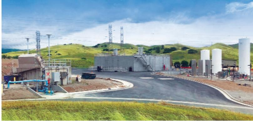
project included the modification of existing facilities and construction of new facilities including an ozone generation building, contactor structure, existing filters modifications, chemical feed facilities, Power and Water Resource Pooling Authority (PWRPA) electrical facilities and a plant utility water pump station. This project improves water quality, enhances the water treatment process, and increase water production reliability.
