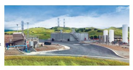
project included the modification of existing facilities and construction of new facilities including an ozone generation building, contactor structure, existing filters modifications, chemical feed facilities, Power and Water Resource Pooling Authority (PWRPA) electrical facilities and a plant utility water pump station. This project improves water quality, enhances the water treatment process, and increase water production reliability.
