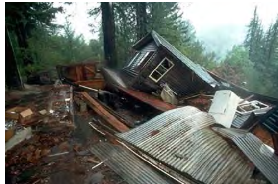
House moved off cement foundation
