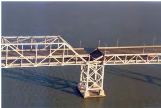
Collapsed San Francisco- Oakland Bay Bridge
