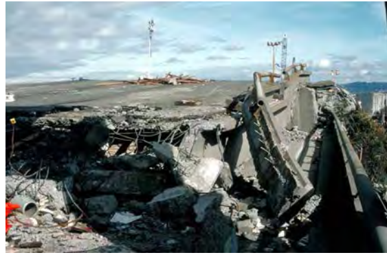
Collapsed Cypress viaduct
