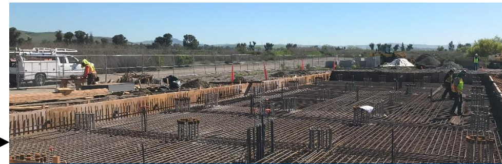
Chain of Lakes PFAS Treatment Plant Constructing Tank Pad, April 2024
