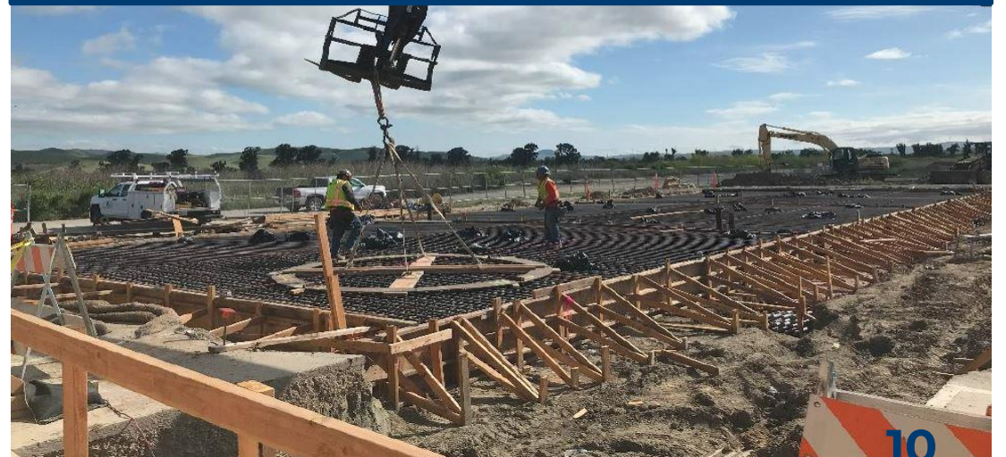
Construction of Chain of Lakes PFAS Treatment Facility
