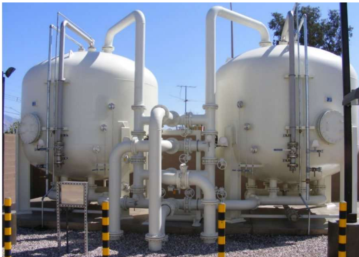
Figure 4 Example Pressure GAC Adsorption Lead-Lag Pressure Vessels
