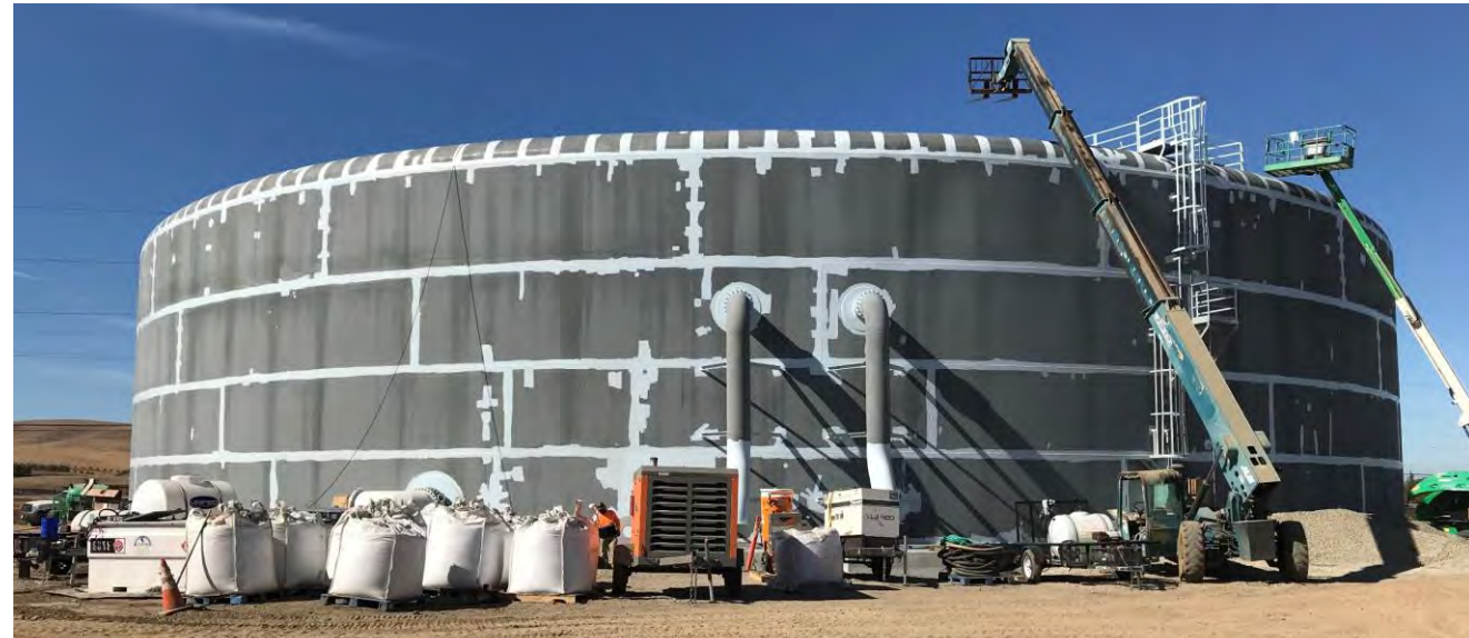
Exterior Coating (starting with seams and roof) – 7/8/21
