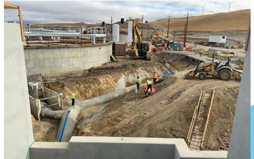
Backfilling 48-Inch Settled Water Pipe From Clarifiers to New Filters – 6/14/21
