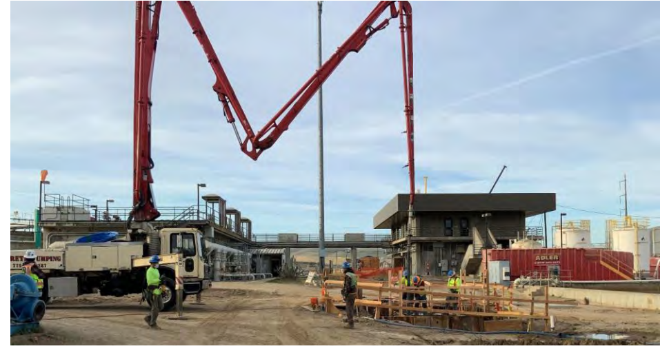
Pouring Concrete for Chemical Vault Construction – 4/20/21
