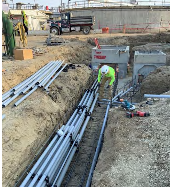
Installing Electrical Conduit to Filter-to-Waste Return Pump Station – 7/14/21
