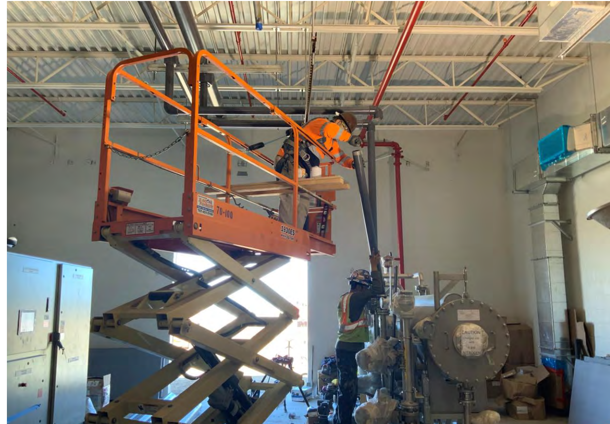
Installing Cooling Water Pipes – 5/5/21
