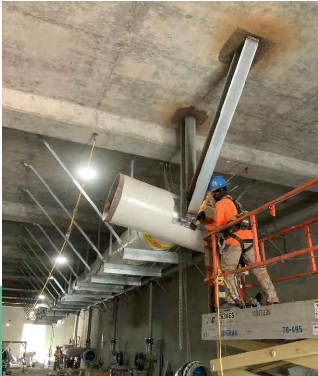
Installing 24-Inch Backwash Pipe in Filter Pipe Gallery – 5/5/21
