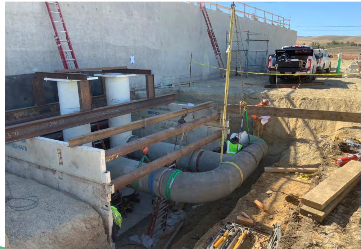
Installing Piping at Filter-to-Waste Return Pump Station – 4/27/21
