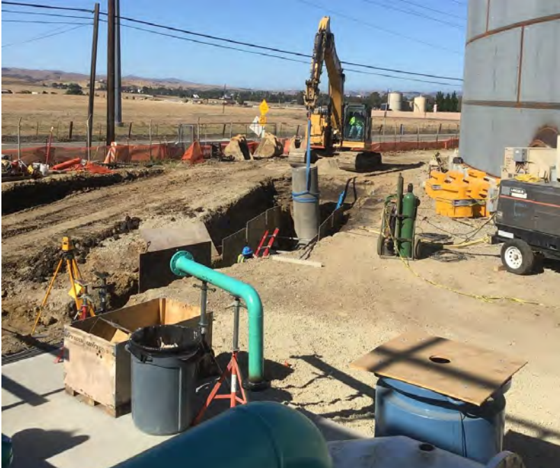
Installing 36-Inch Treated Water Pipe from TWMV to 5 MG CW – 5/18/21
