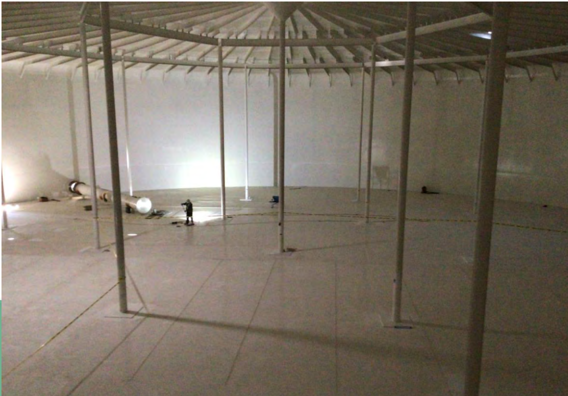
Touching Up Interior Coating of 5 MG Clearwell – 5/27/21
