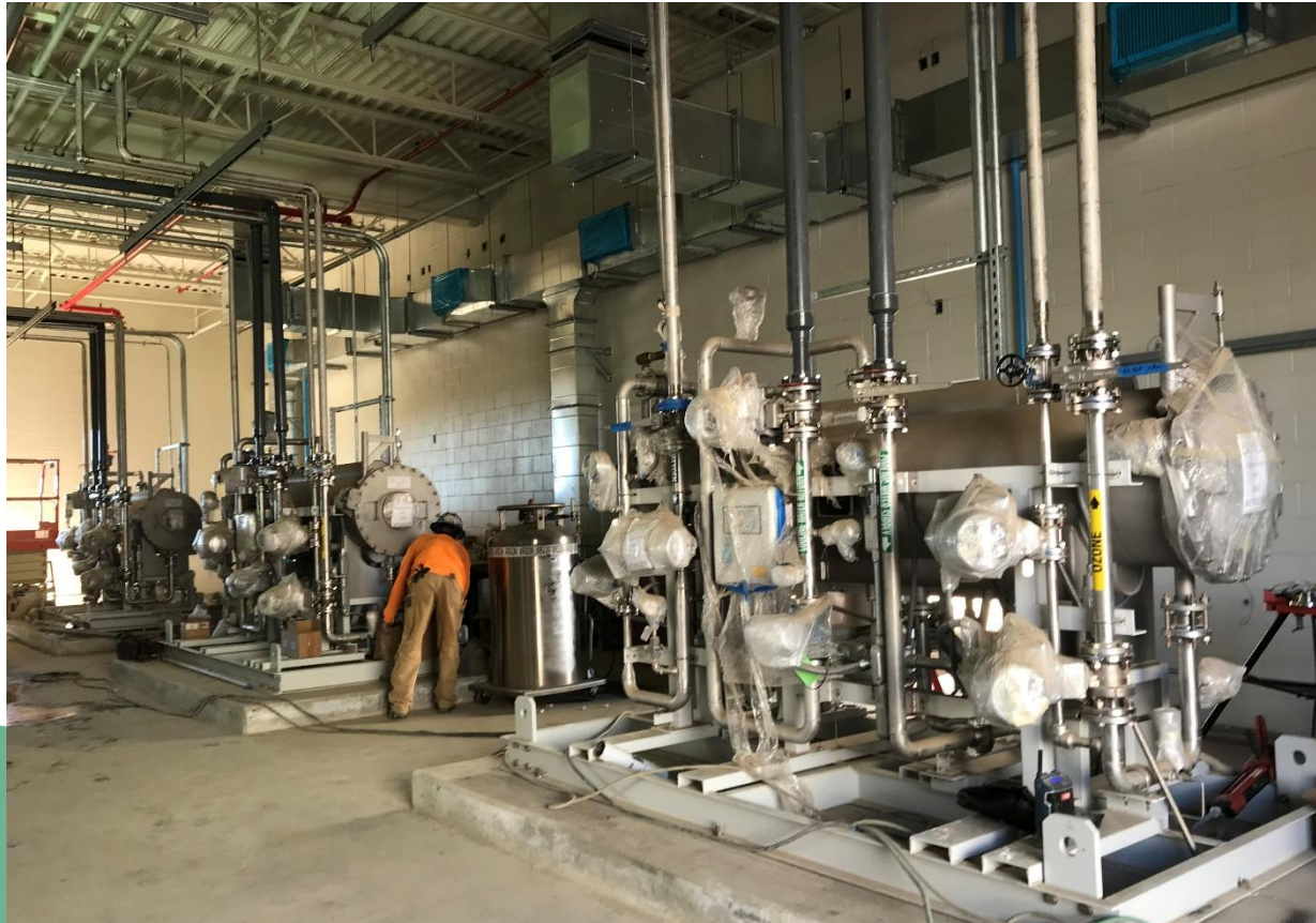
General View of Ozone Generation Building – 9/27/21
