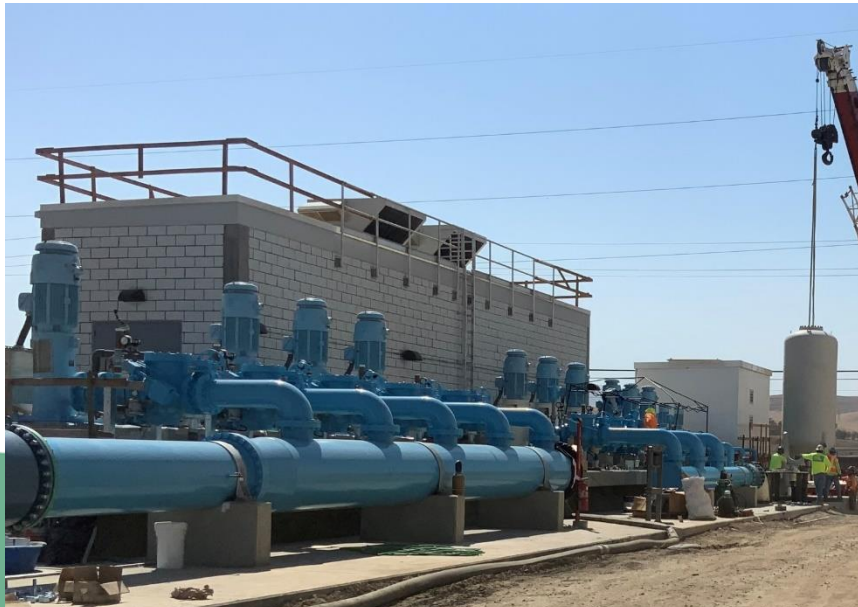
General View of Treated Water Pump Station – 9/17/21
