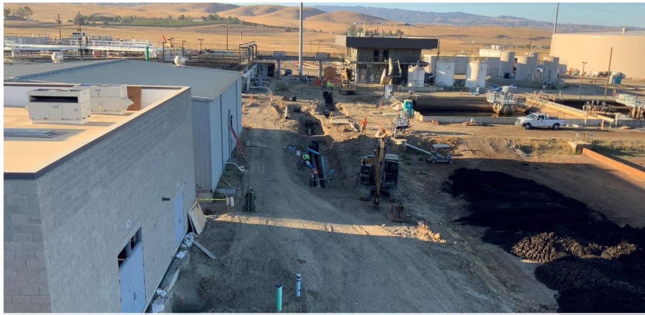
Excavating Chemical Duct Bank – 9/14/21
