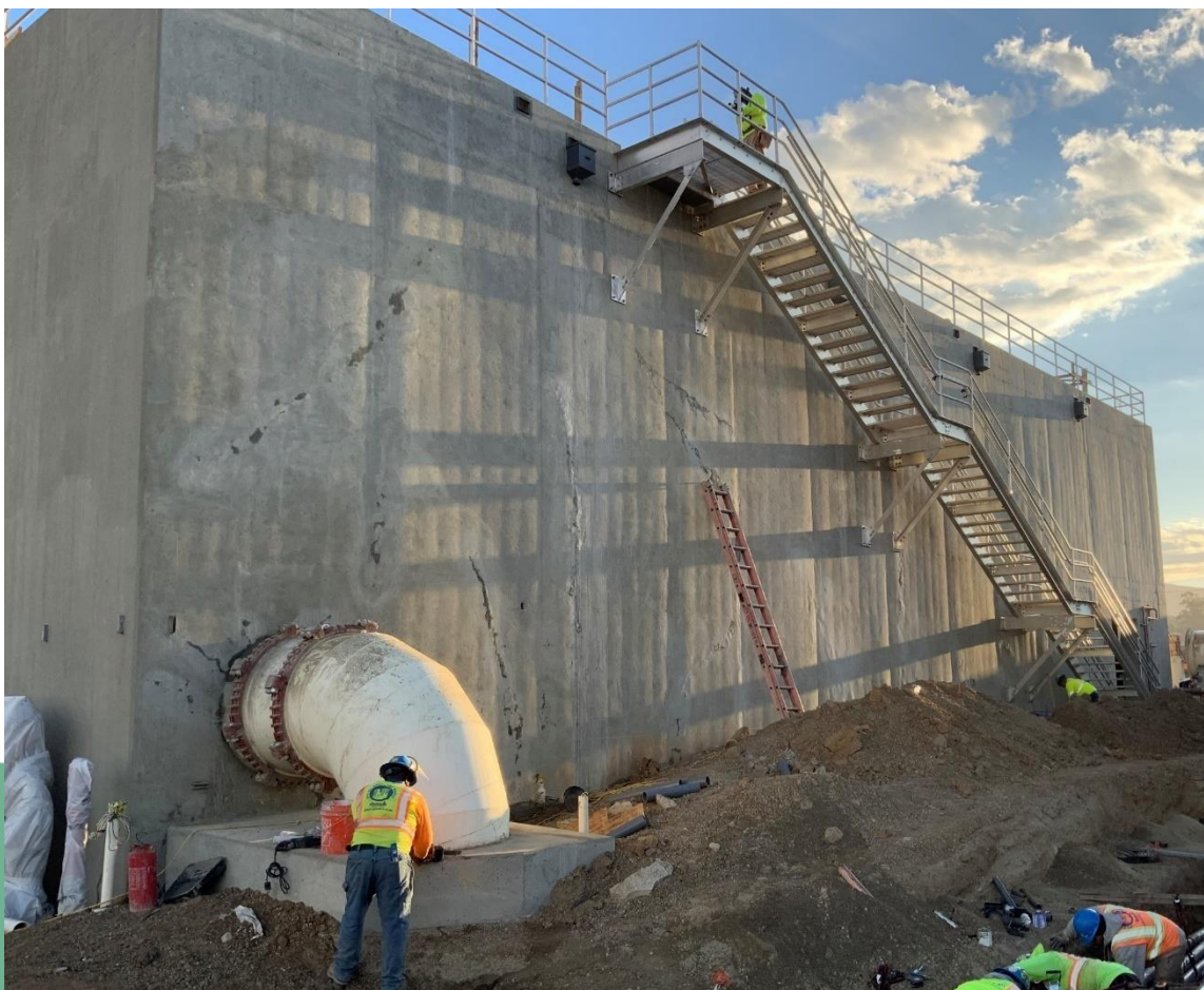
General View of Ozone Contactor Structure – 9/10/21
