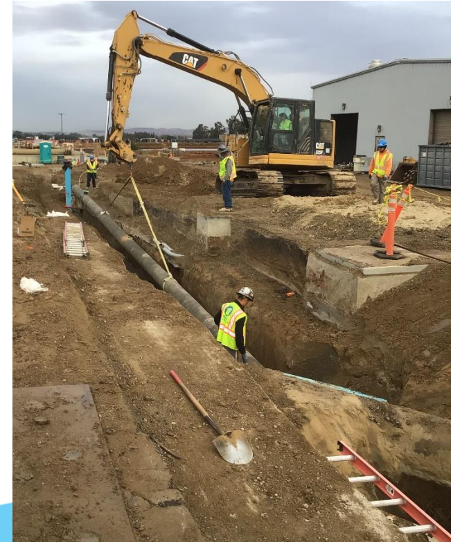
Installing Plant Water Piping – 10/21/21
