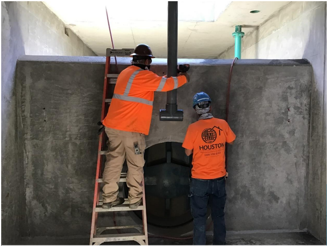
Installing Sodium Hypochlorite Injection Diffuser – 9/15/21
