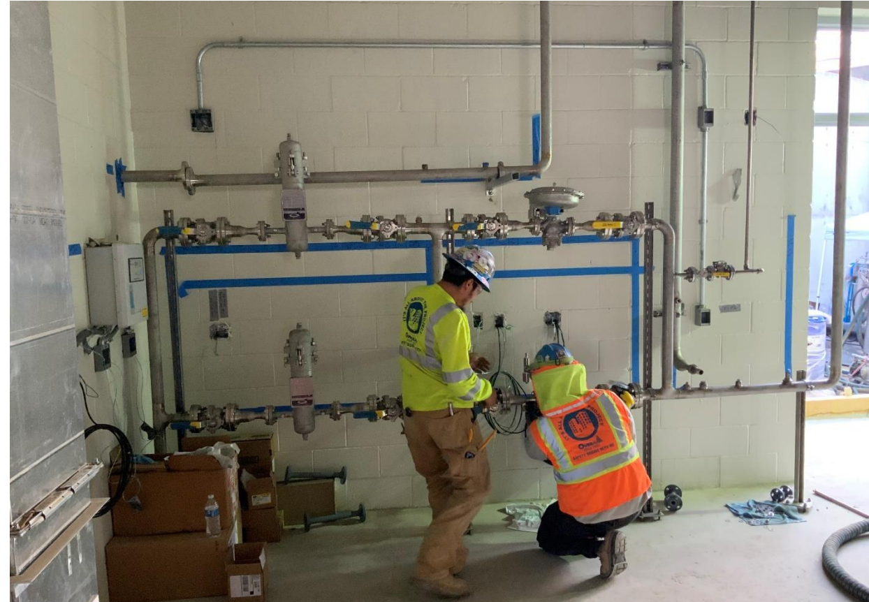
Installing Valves and Gauges on Ozone Piping – 10/5/21
