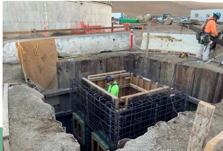
Constructing Chemical Containment Vault – 9/20/21
