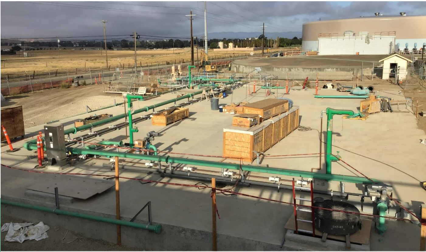
General View of Deck of Chlorine Contact Basin – 8/4/21
