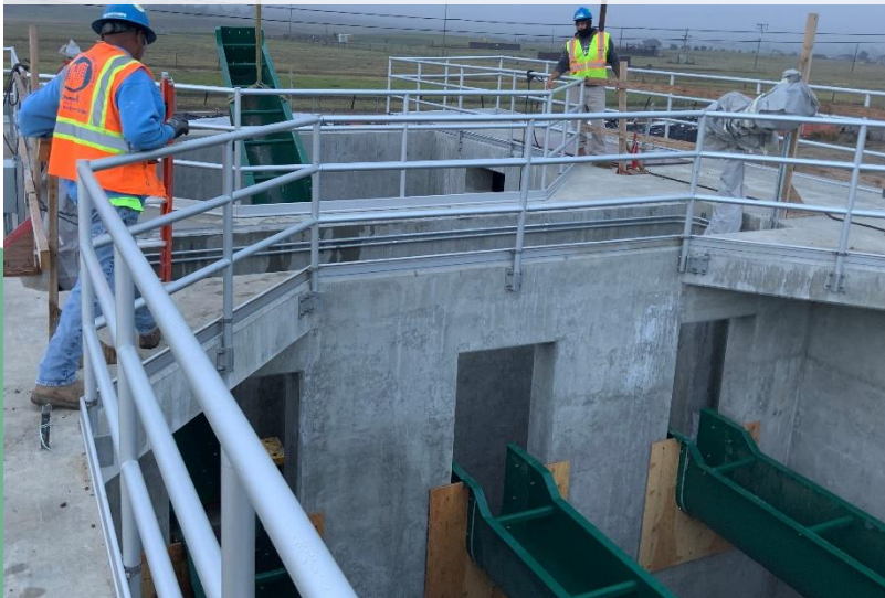
Installation of Filter Troughs – 11/2/21
