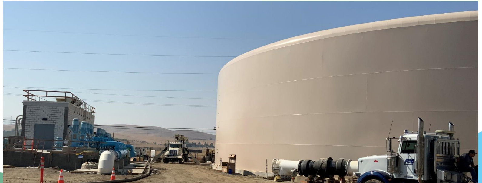
General View of 5 MG Clearwell and Treated Water Pump Station – 9/3/21
