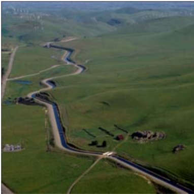
Supply from the SWP is delivered via the South Bay Aqueduct, which can also be used to deliver other supplies.
