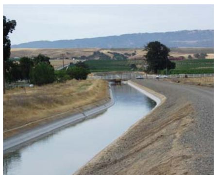
South Bay Aqueduct (at Tesla Road)
