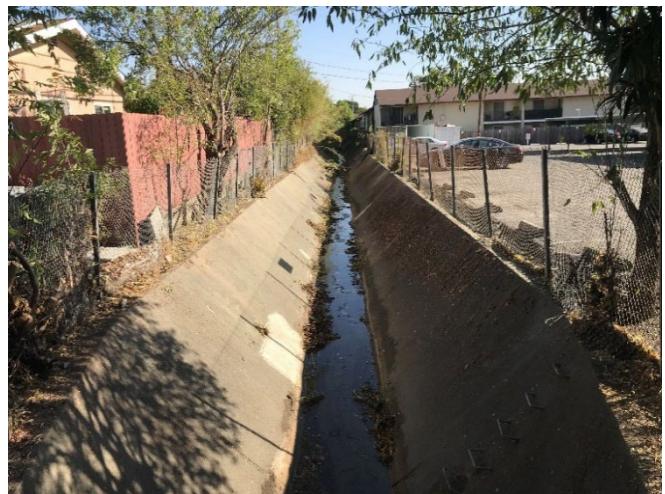
Figure 8. Typical concrete-lined channels requiring repair, rehabilitation, or replacement
