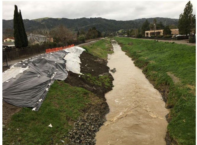
Figure 11. Slope failure (left) and emergency repairs (right) along Arroyo Mocho channel during 2017 storms
