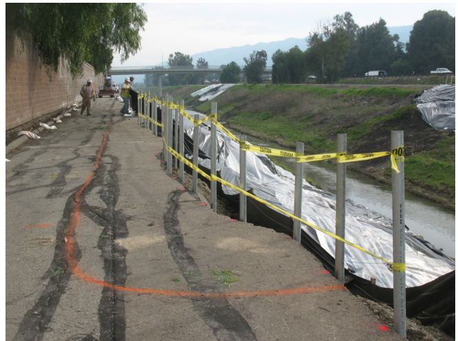
Figure 12. Sewer main pipeline erosion (left) and emergency repair (right) along Alamo Canal and Arroyo de la Laguna channels during 2017 storms
