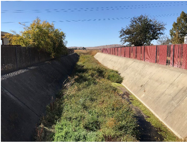
Figure 7. Vegetation growth and sedimentation accumulation in Altamont Creek channel, Line R (left), and vegetation growth including invasive species ( Arundo donax ) in Alamo Creek channel, Line J (right)
