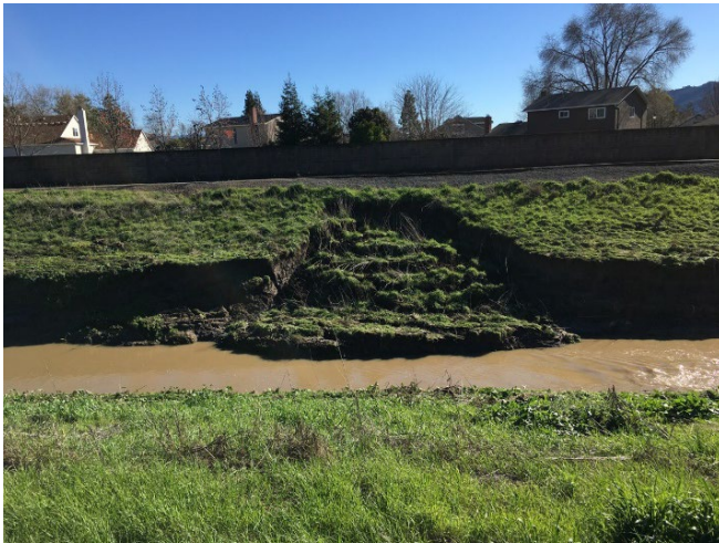
Figure 11. Slope failure (left) and emergency repairs (right) along Arroyo Mocho channel during 2017 storms
