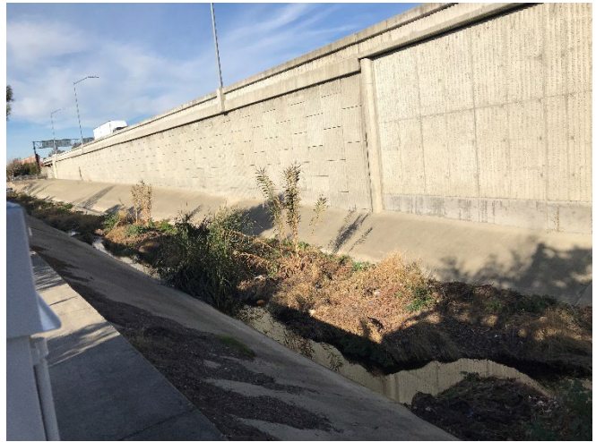
Figure 7. Vegetation growth and sedimentation accumulation in Altamont Creek channel, Line R (left), and vegetation growth including invasive species ( Arundo donax ) in Alamo Creek channel, Line J (right)
