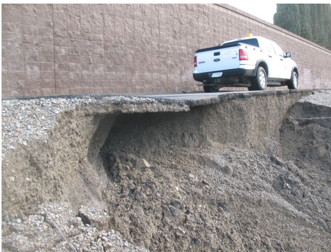
Figure 12. Sewer main pipeline erosion (left) and emergency repair (right) along Alamo Canal and Arroyo de la Laguna channels during 2017 storms
