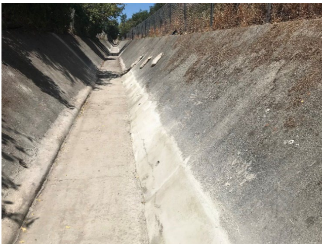
Figure 8. Typical concrete-lined channels requiring repair, rehabilitation, or replacement
